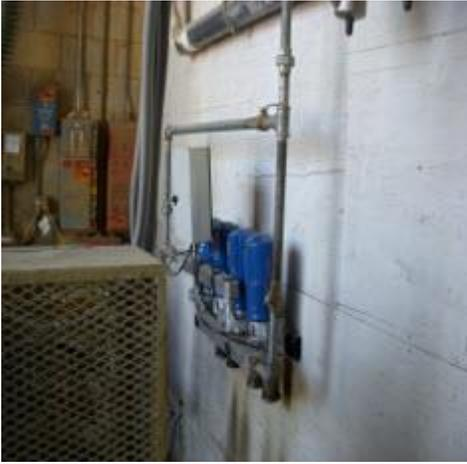
Commonly used in conjunction with large air compressors and systems or offering the capability to mount directly on small compressors, is engineered to dry compressed air directly from a compressor's reservoir tank or at a point of use. This eliminates the need for after coolers and, in most cases, additional external filters and any other corollary equipment. A molecular sieve (desiccant) and filters are housed within spin on/off cartridges.
